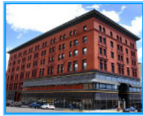
Facilities Offices and Laboratories Butte, Montana
